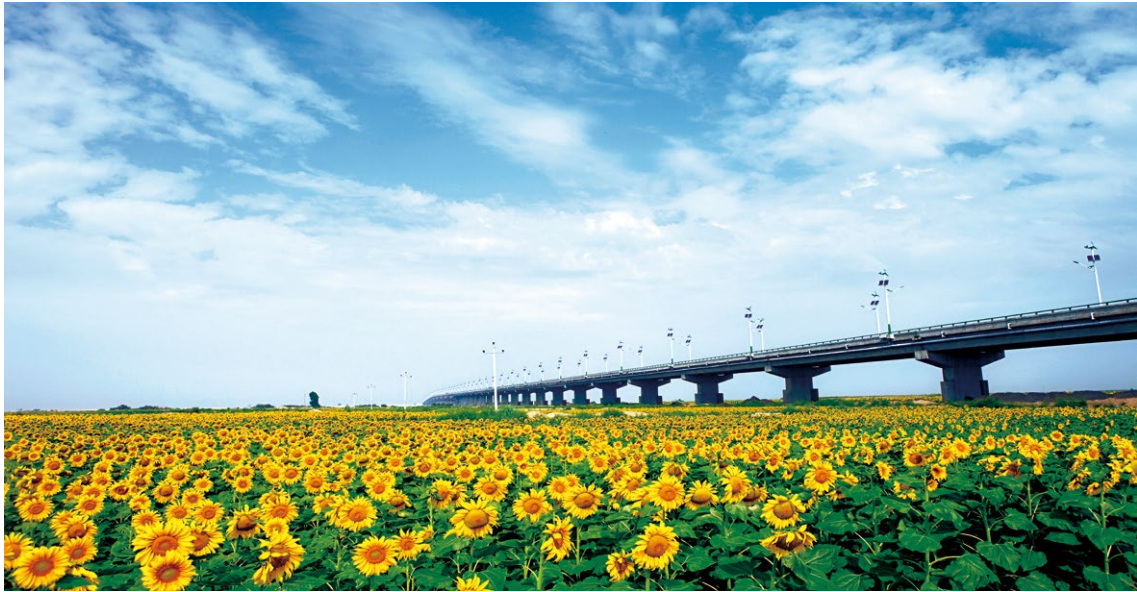
Figure 5.1. Yellow River highway.
