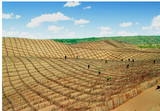
Figure 4.4. Sand barrier technology using a grid pattern of bundled Salix (willow) stems, crop straw and other materials.
